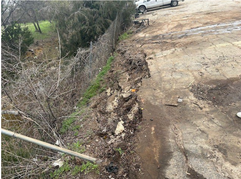
Part of Problem Area 3 Improvements.
